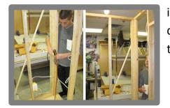
Students began the semester building a 4x6 room where they learned to build walls properly, build walls with a door, install power for outlets and switches for lights.
