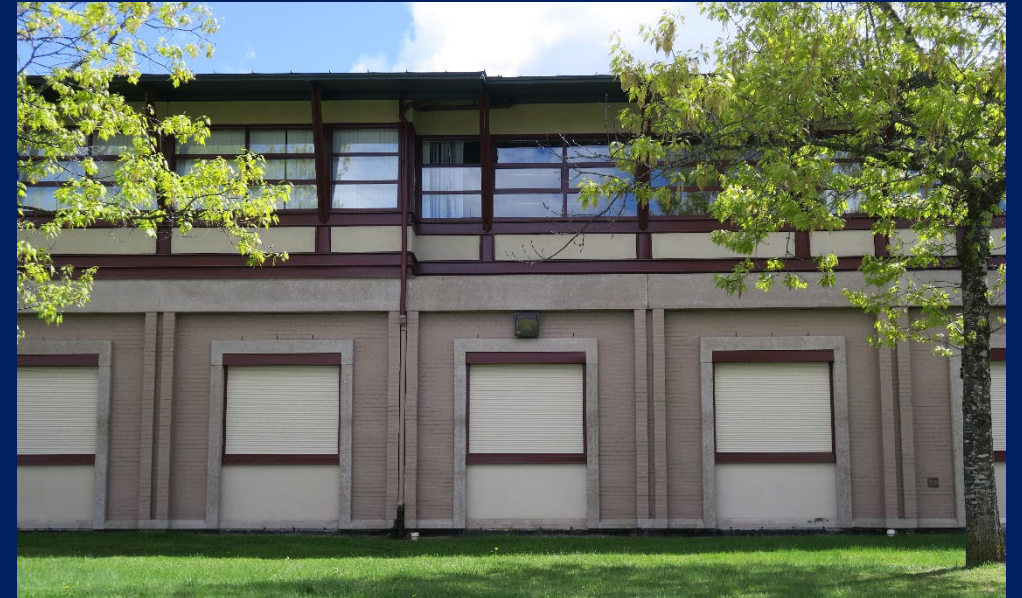
Tamanawis Secondary School Addition (Site 150)
