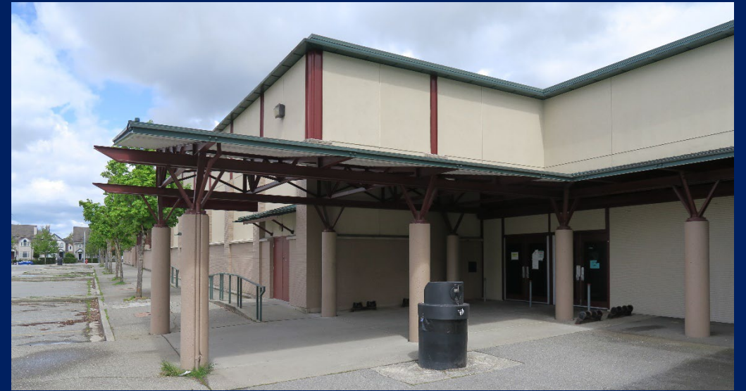
Tamanawis Secondary School Addition (Site 150)
