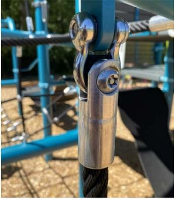
**Aluminum Net Connectors:** All climbing net connections are made with metal parts that stand the test of time. Beware of plastic connectors that break down in UV light and the dynamic stresses created by flexible cable. For longevity, all dynamic cable play should connect to the structural framework via a flexible connection. This prevents the cable from “paper clip” fracturing.
